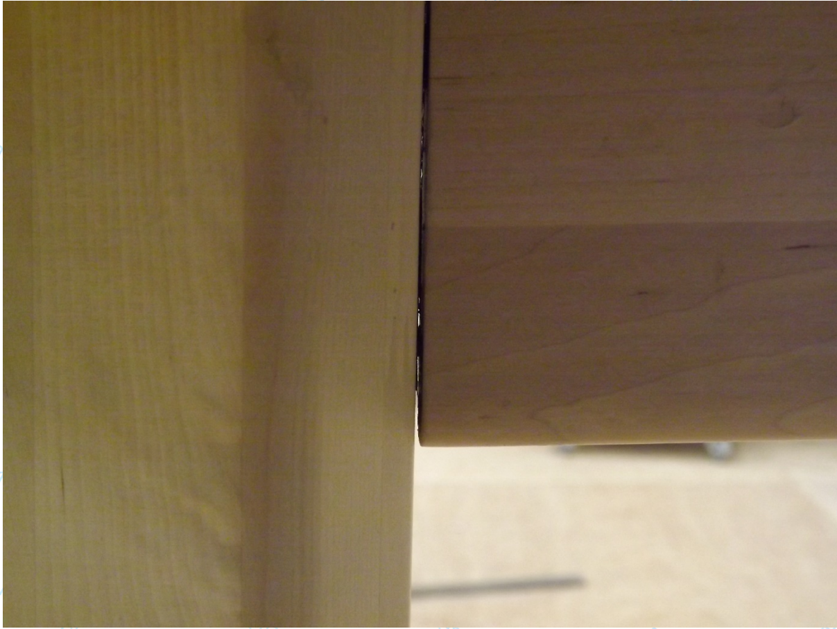
Picture 3: Slight loosening of joint of the 'Rock Table'
